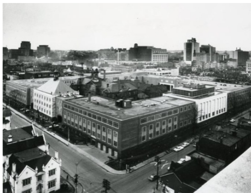
Figure 6: Kerr Hall archival photograph [27].
