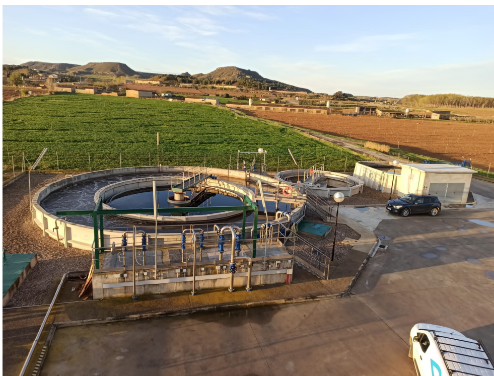
Figure 1: Binaced WWTP (Huesca, Spain).
