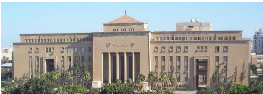
Figure 3: The Engineering Faculty building at Alexandria University [8].
