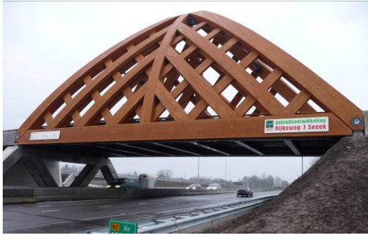
Figure 3: A large scale application of Accoya® wood – Sneek bridge, the Netherlands. The first ever heavy traffic road bridge with a wooden load bearing structure with an anticipated lifespan of 80 years.
