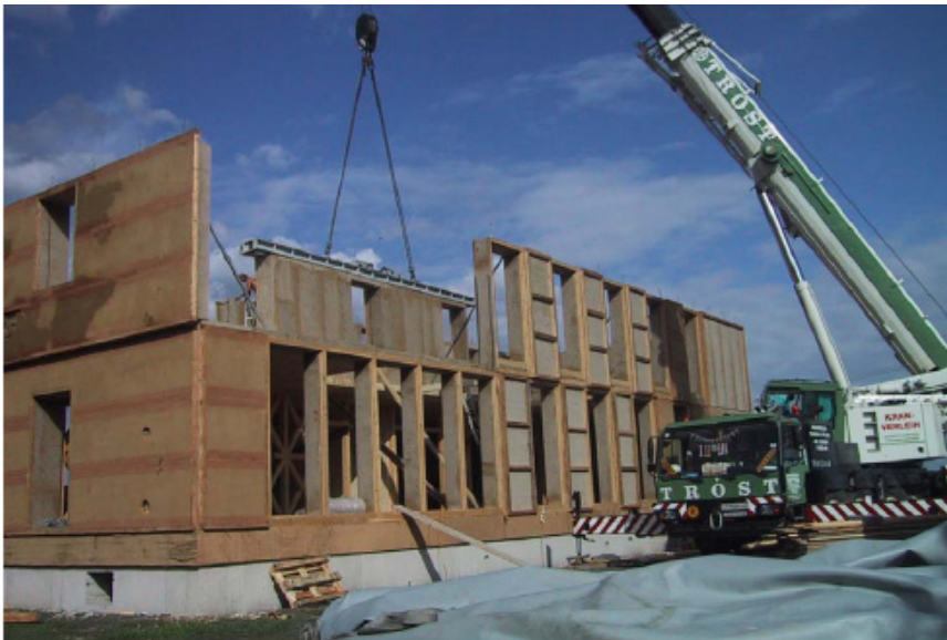
Figure 5: Office building Tattendorf, construction of south facade [17].
