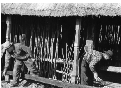
Figure 8: Vertical wattle and timber, Dumbrăveni.
