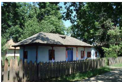
Figure 6: Grange from Rușețu Buzău County in “DG”NVM.
