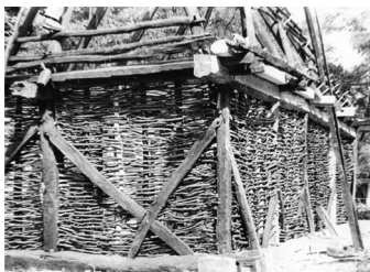
Figure 4: Horizontal wattle and timber, Dumitra.
