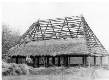
Figure 9: The building of the roof, Dumbrăveni.
