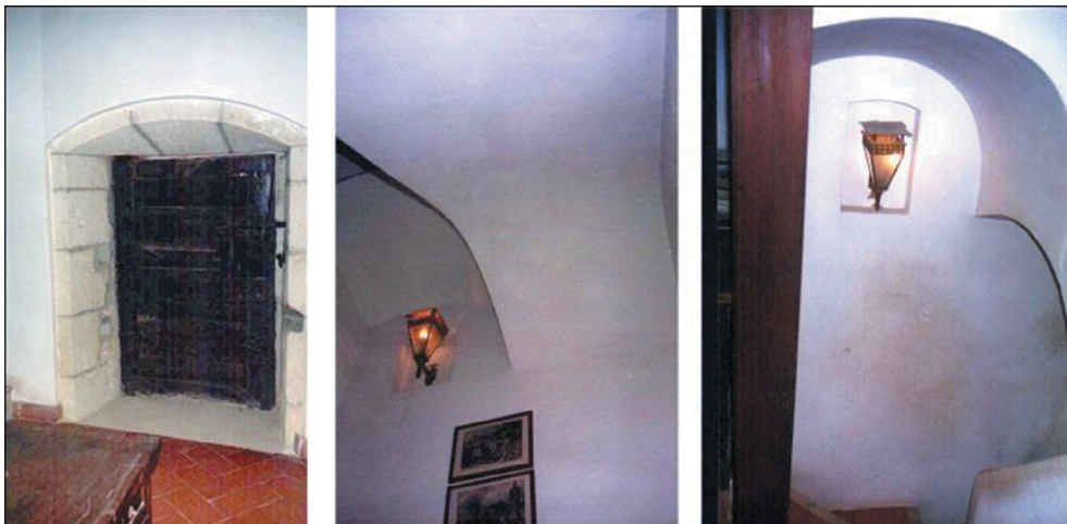
Figure 4: Left – communication door of the house and tower located on the first floor. Center and right – slab staircase.
