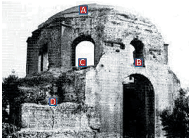
Figure 4: Measurement points on the façade.
