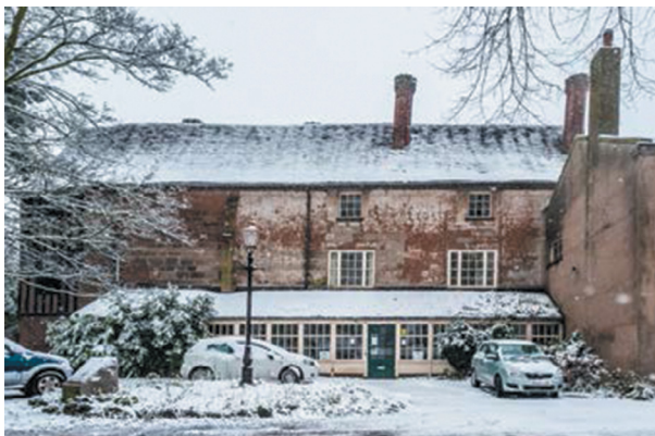
Figure 3: The Charterhouse, west façade.
