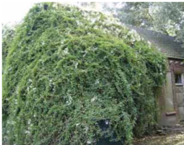
Figure 10: Example of possible damages due to the lack of maintenance: direct green facade with climbing plants.
