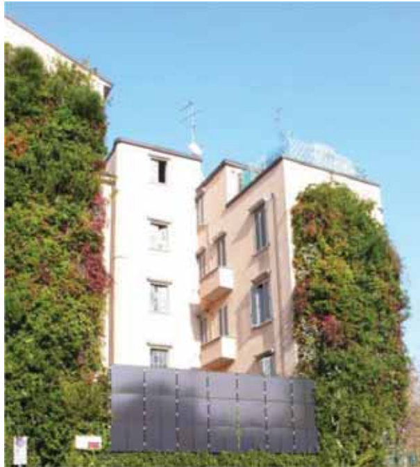
Figure 3: Green wall designed by Temprano in Milan (Italy).
