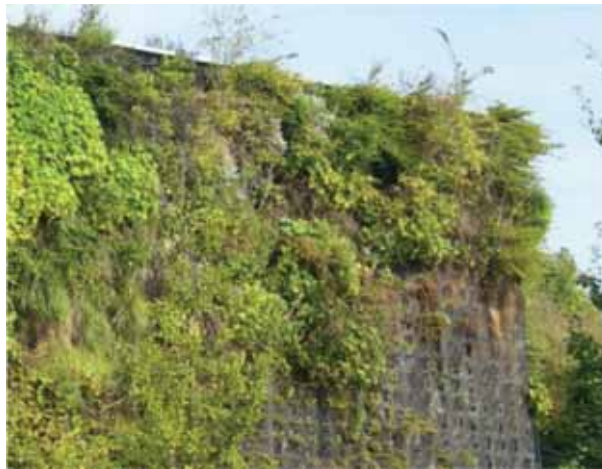
Figure 9: Example of possible damages due to the lack of maintenance and to design mistakes: living wall system based on felt layers in Amsterdam.
