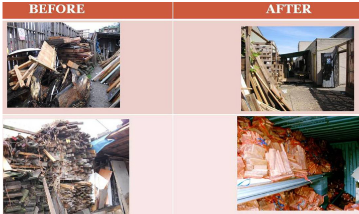
Figure 1: Before, the worksite was hard to access, dangerous and materials uncategorised. Since, a roof shelter has been provided, shelving and items are categorised and logged in an inventory and can be easily accessed for reuse.
